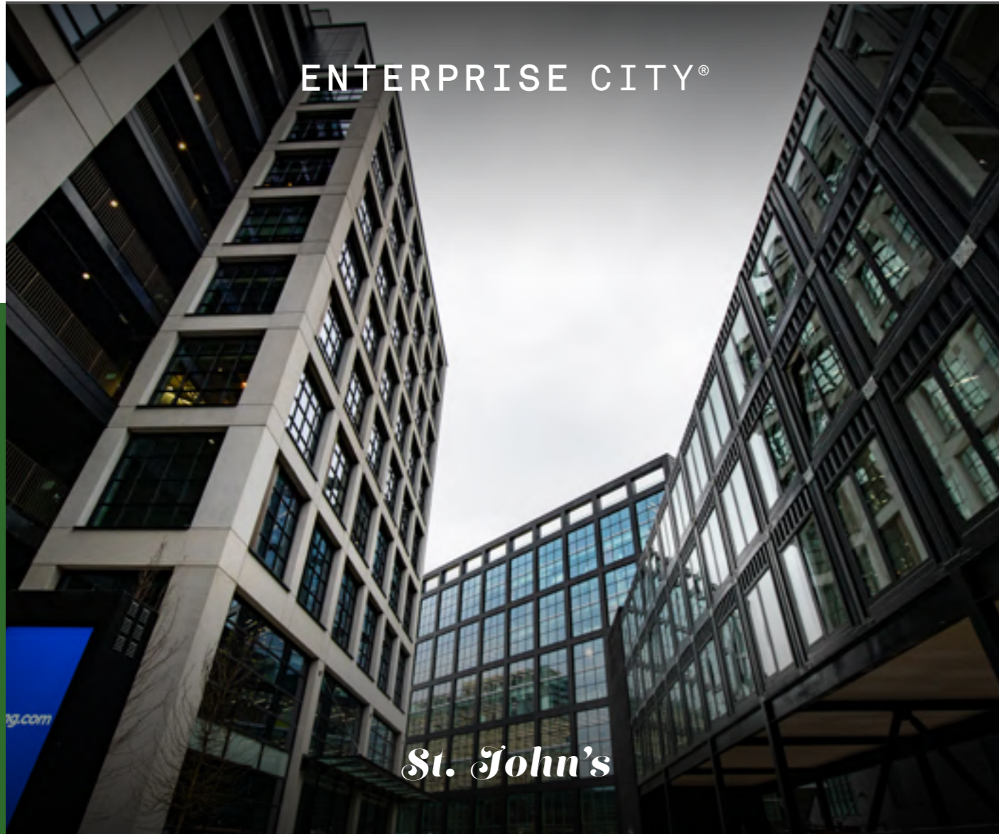
Progress at St. John's, February 2023. MGY on the left, Cube Space on the right with the Globe building at the back.
